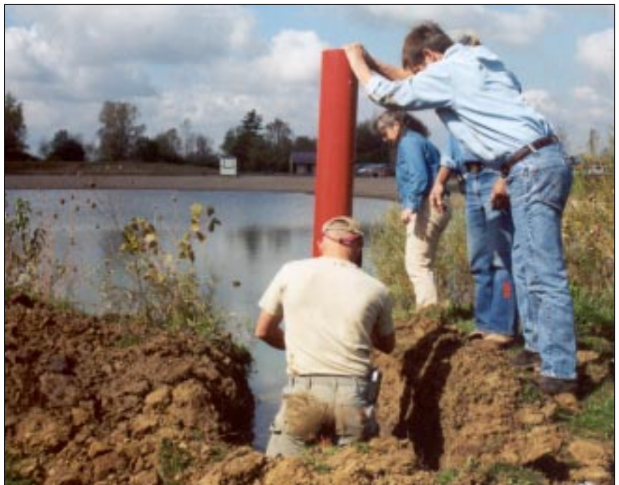
Bart Bales and Tom Fisher finish a dry hydrant demonstration installation at Johnson County Park.
